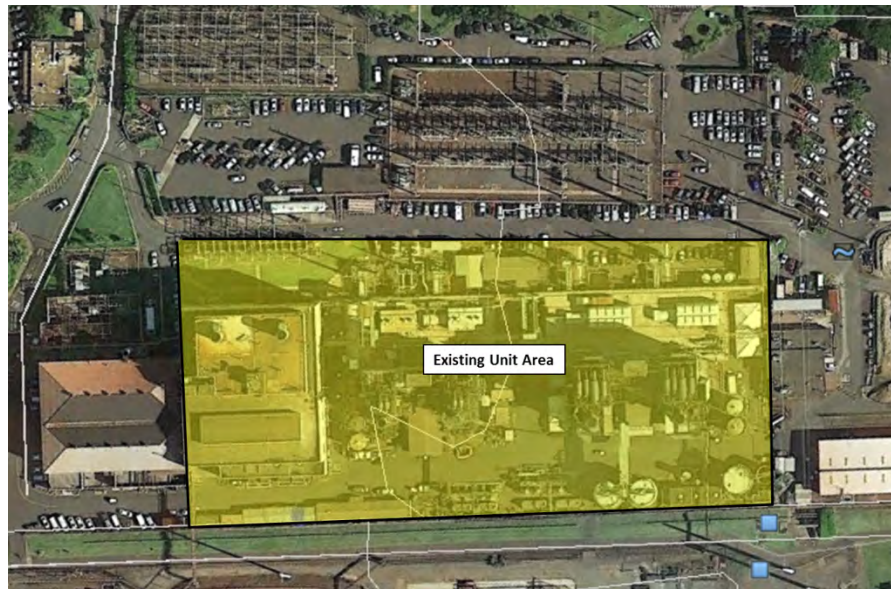
Figure 5-14. Existing Waiau Generating Unit Area
